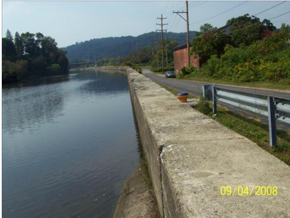
Figure 6.6-3: Concrete Wall along Canal
