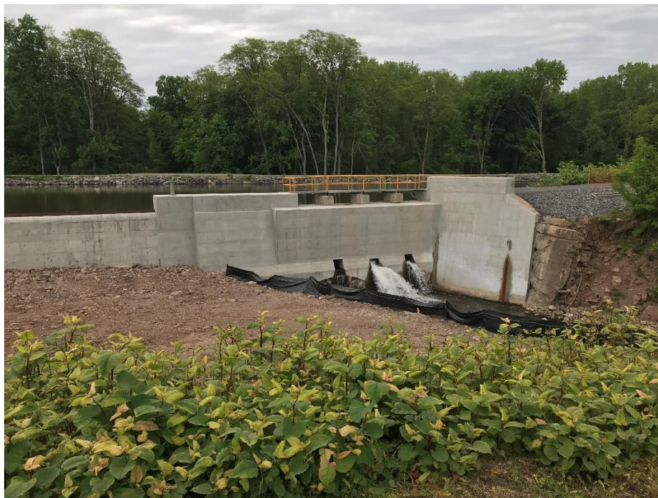
Figure 6.6-2: Erie Canal Waste Weir (and Sluice Gates) at Albion, NY
