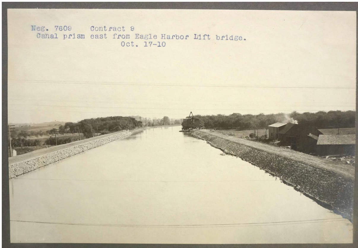
Figure 3.9-2: Historic View of Canal at Eagle Harbor Waterport Road, Orleans County, NY
