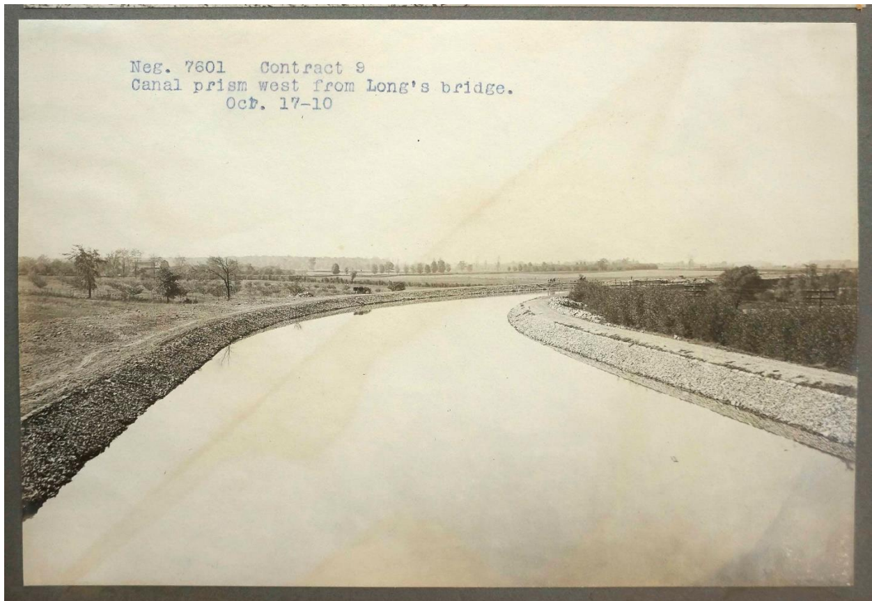
Figure 3.10-1: Treeless Earthen Embankments During the Period of Significance
