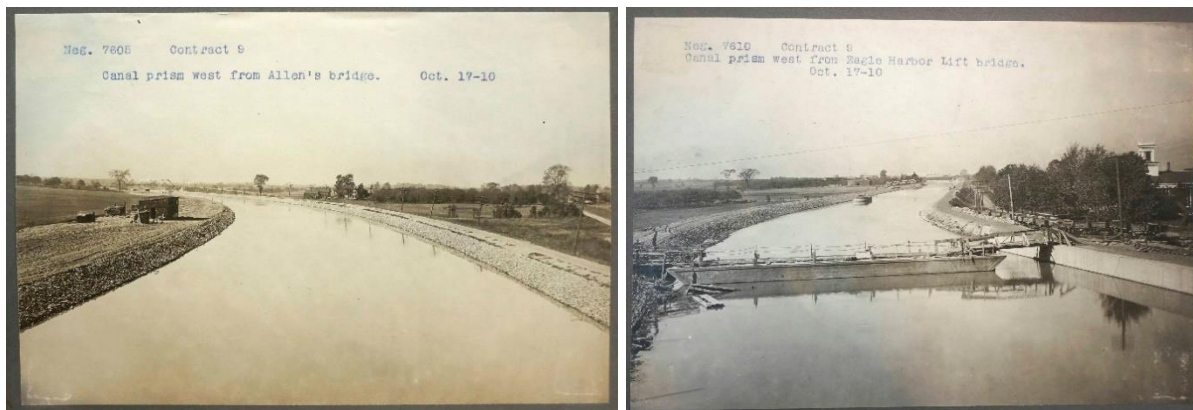
Figure 3.2-1: Historical Photos of Canal at Allen's Bridge and Eagle Harbor Bridge
