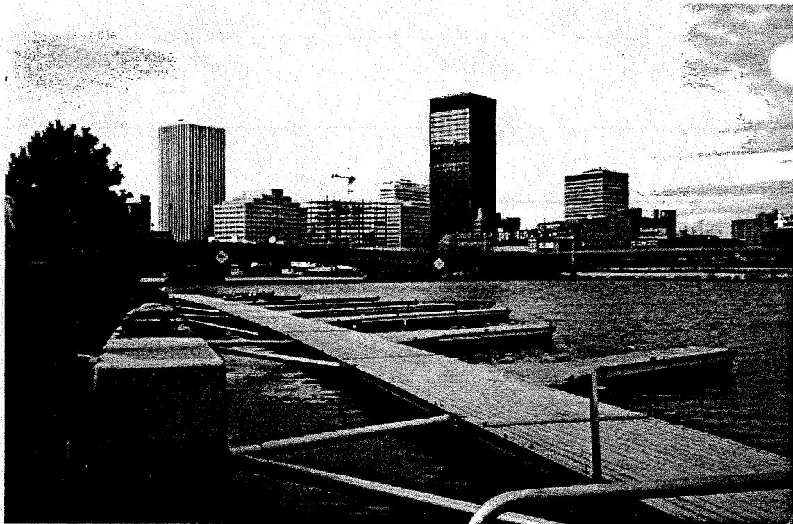
View looking northeast at the I-490 bridge and down- town Rochester.
