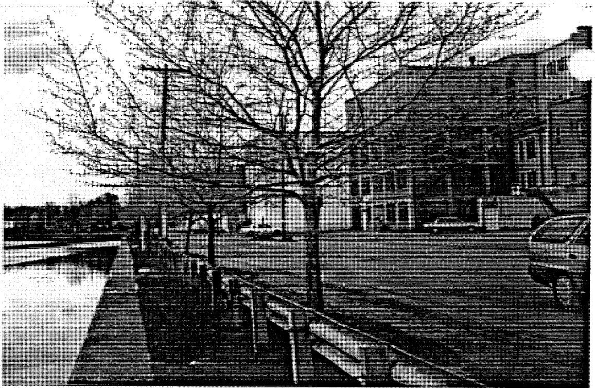
View looking west along the terminal wall.
